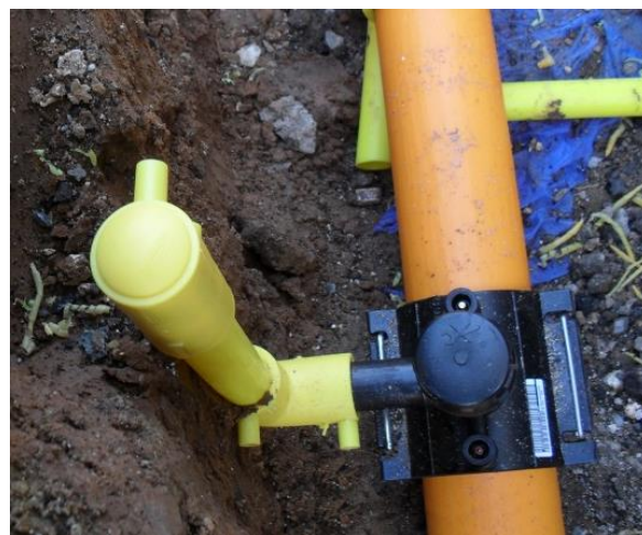
Fig. 12 – photo of a capped purge point as it is no longer required
