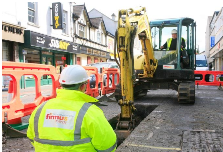
Fig. 2 – photo showing the traditional open cut technique
