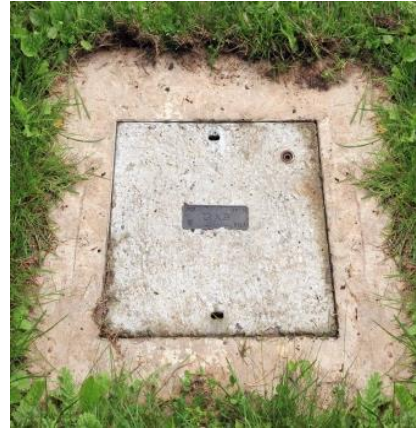
Fig. 8 – photos showing a cast iron and concrete gas toby lid
