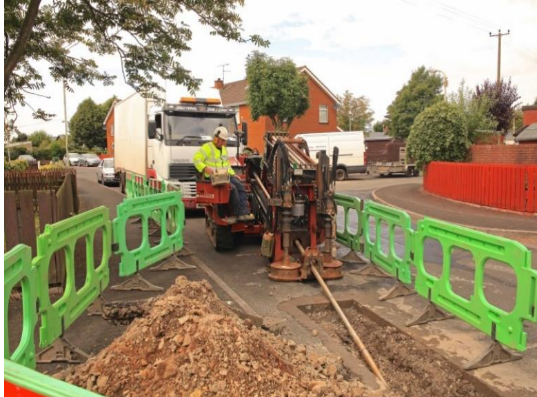
Fig. 3 – photo showing directional drilling technique
